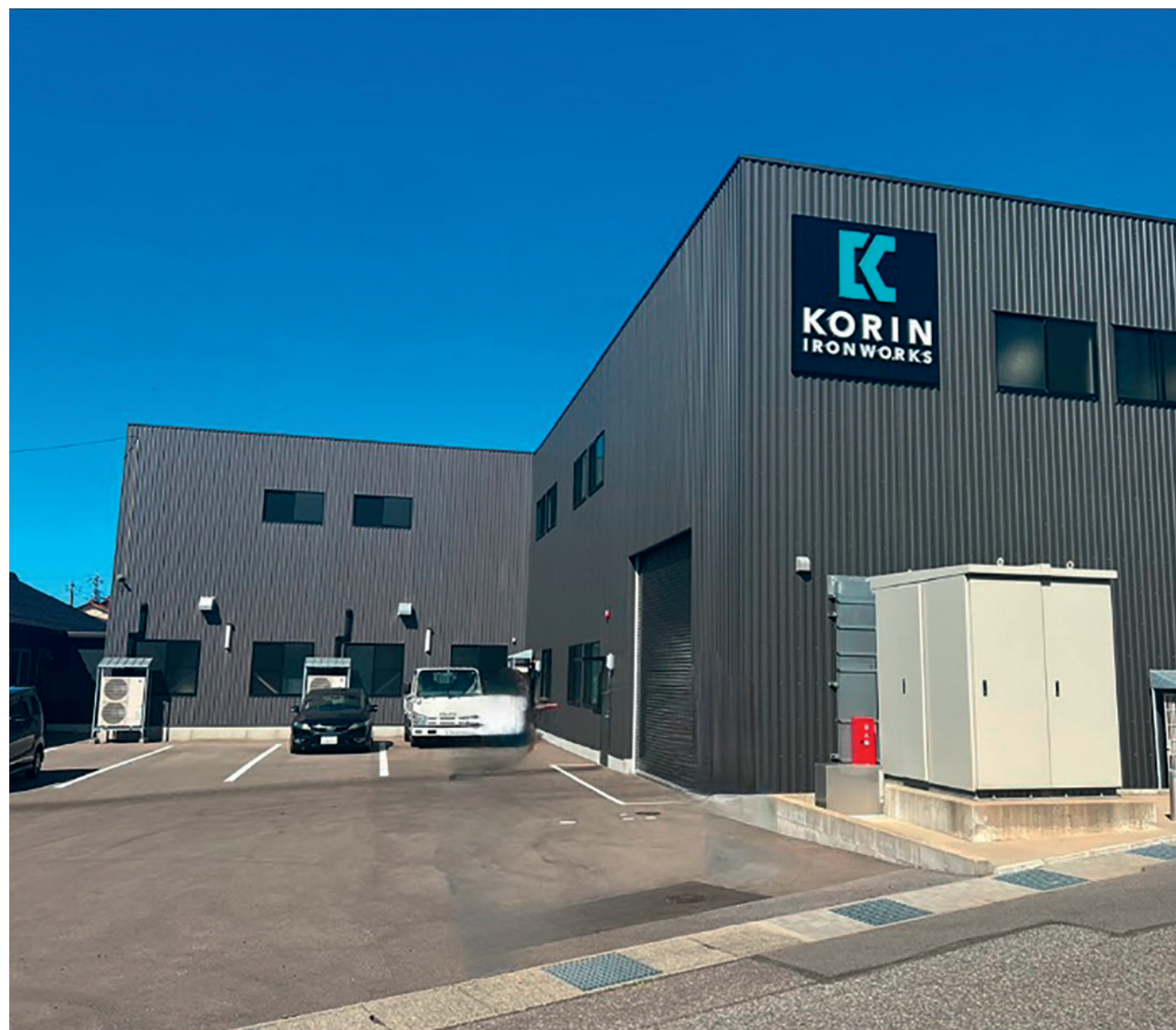
Newly built factory of Korin Iron Works
